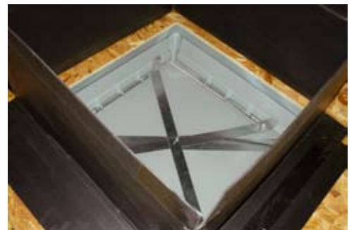
(Top view of inlet from the attic.)
